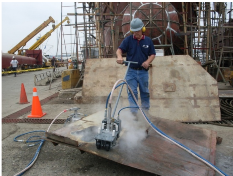
Figura No. 5 Hydroblasting
